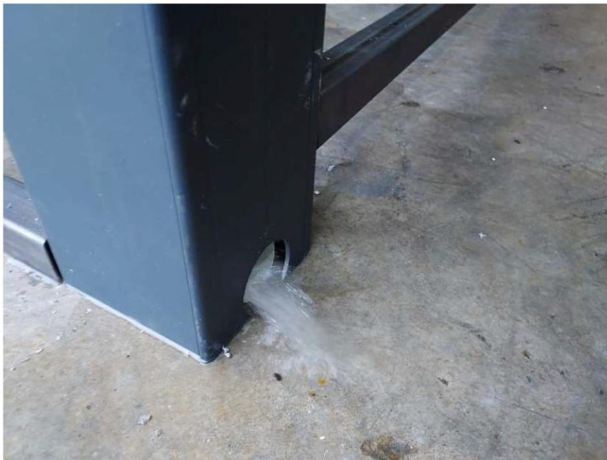
Photo 4. View of the drainage system during the watertightness test.
